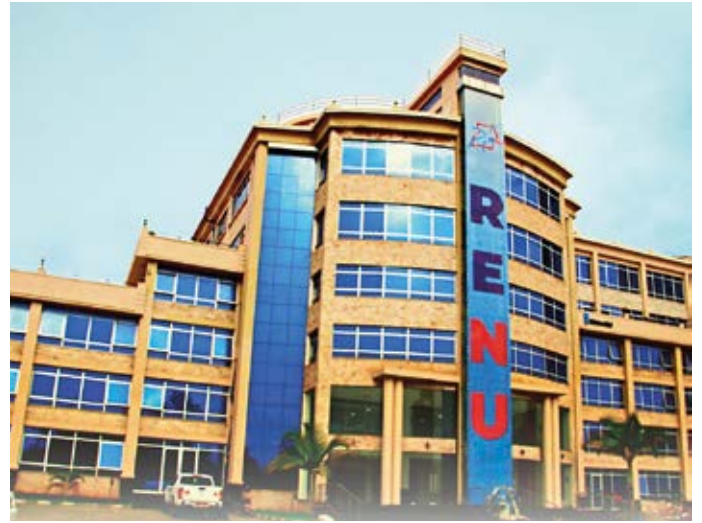
RENU's new office premises at Plot 6, Mabua Rd, Kololo, Kampala
